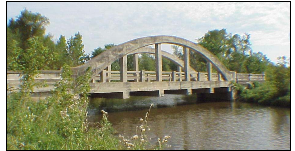
6.3.9 Above: Concrete-arch bridge spanning the Seine River at Ste. Anne Constructed in 1921 and known locally as the 'Piney Road Bridge', this structure was designated a municipal heritage site by the Rural Municipality of Ste. Anne in July 1987, and was the first bridge in Manitoba to be designated a heritage site. It is the only surviving concrete arch bridge in southeastern Manitoba. (Photo: Historic Resources Branch.)
