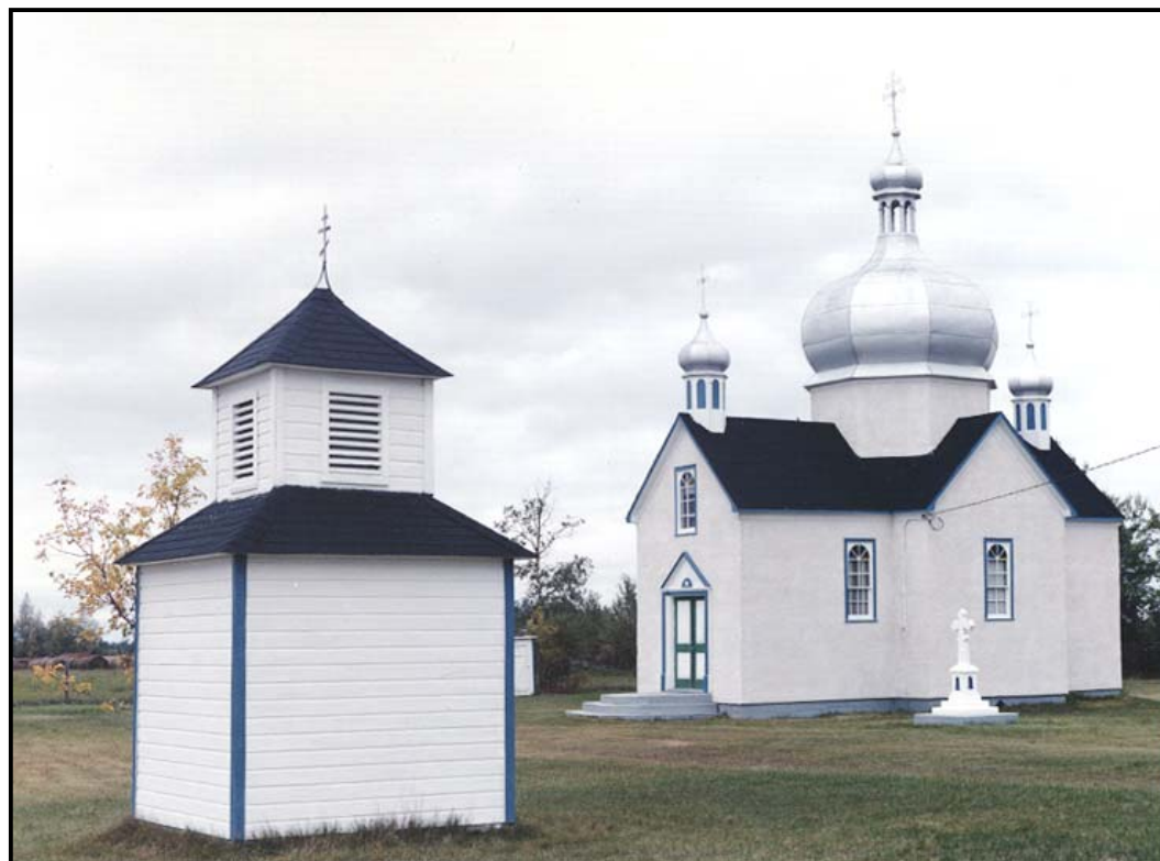
5.5.5 Above: St. Nicholas Ukrainian Greek Orthodox Church, Arbakka district Erected in 1939, the asphalt roofing and stucco exterior finish are typical construction materials for the period; while the cruciform plan, multi-domed roof are traditional design elements. The stand-alone bell tower is characteristic of all Ukrainian churches and although strictly utilitarian, they often feature unusual and attractive designs. (Photo: Historic Resources Branch.)
