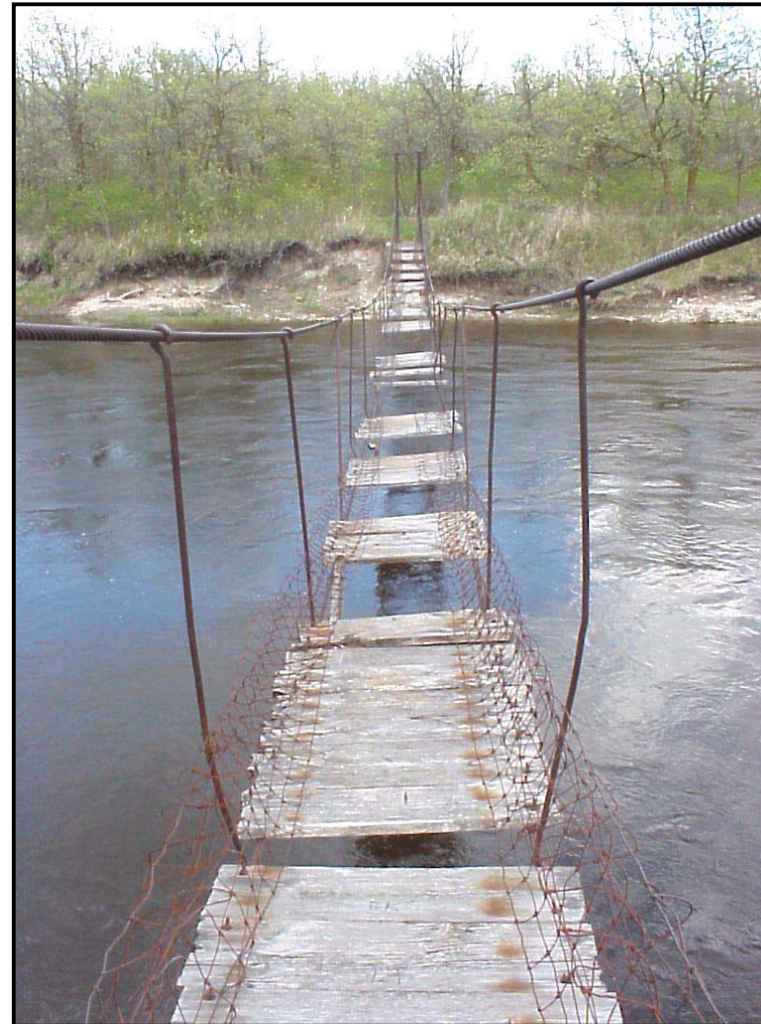
6.3.8. Above: The Senkiw School Suspension Bridge One of only a handful of suspension bridges remaining in Manitoba, this structure was constructed around 1934 by area residents using old agricultural equipment components. It replaced an earlier cable-car apparatus which area school children used to cross the Roseau River to attend the nearby Senkiw School. Designated a municipal heritage site by the R.M. of Franklin in February 2002, there are plans for its rehabilitation and incorporation into the Trans Canada Trail which passes through the study region. (Photo: Historic Resources Branch.)
