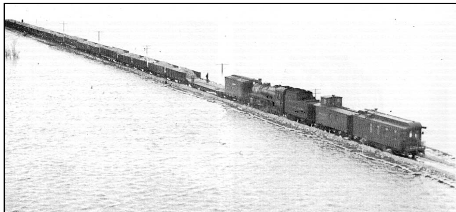
6.2.1 Above: Pembina Branch during the 1950 flood
