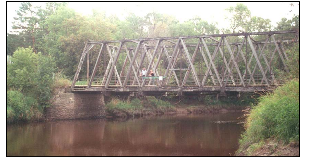
6.3.10 Above: Timber truss bridge spanning the Roseau River at Gardenton Constructed in 1918, this Howe truss wooden bridge is one of only two surviving examples of this bridge type in the study region. It was designated a municipal heritage site by the R.M. of Stuartburn in February 2002. (Photo: Historic Resources Branch.)
