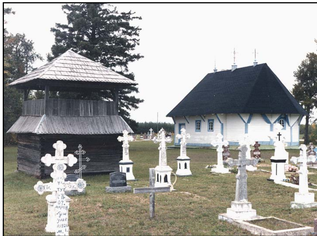
5.5.8 Above: St. Elias Ukrainian Greek Orthodox Church; Sirko Constructed in 1906 of logs, and later sheathed with wood siding, this beautiful and unusual little church is one of only two traditional Bukovynian-style churches remaining in Manitoba. The style is characterized by a steeply-pitched roof, semi-circular ends, and eaves supported by carved cantilevered rafters. Note the original surviving log bell tower. (Photo: Historic Resources Branch.)
